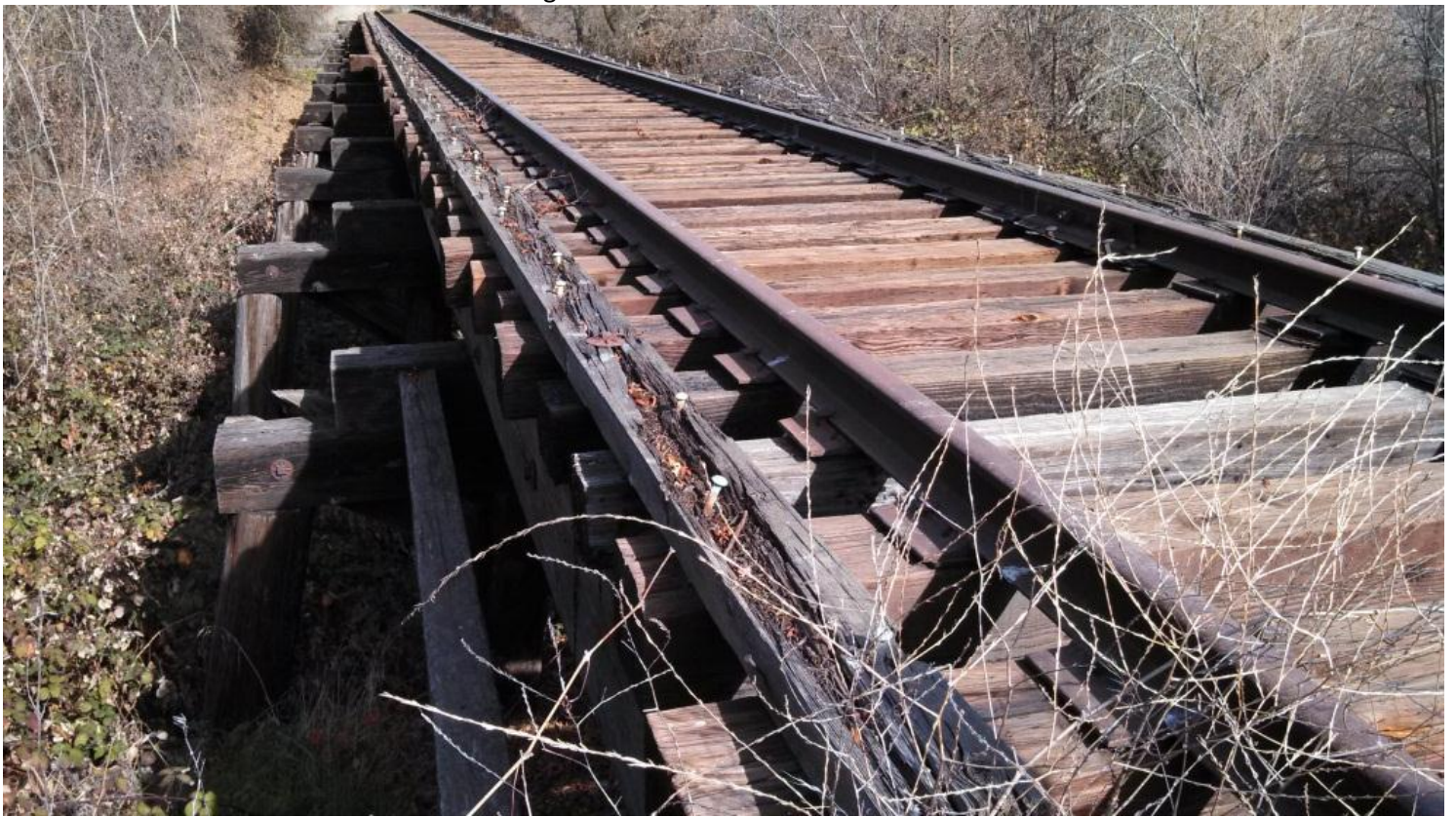
The trestle on the Hood Line.
